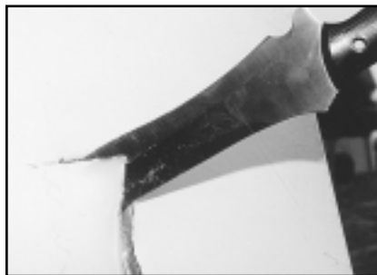
Using the can-opener motion, the author cut an “access hole” in the steel-walled fire door, pulling and prying until the opening was complete.
